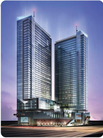
LeCount Towers, New York
