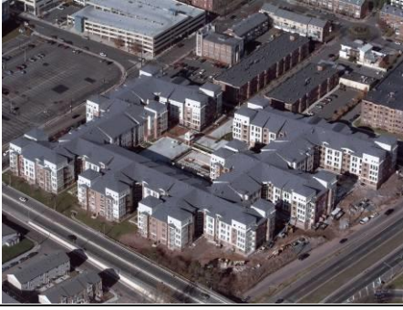
Highland Plaza, New Brunswick, NJ
